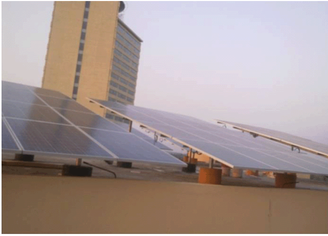
Lulu International Shopping Mall, Coachi. (21 KW Roof Top Solar Power Plant)
