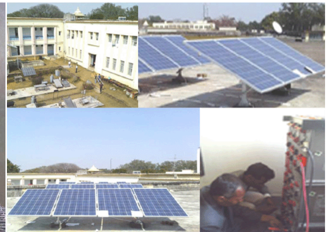
Birla Institute of Technology, Mesra, Ranchi. (3 KW Roof Top Solar Power Plant)
