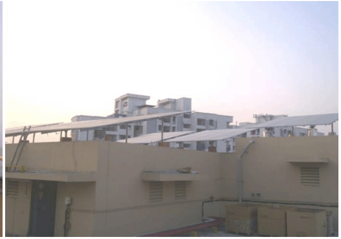
Lulu International Shopping Mall, Coachi. (21 KW Roof Top Solar Power Plant)
